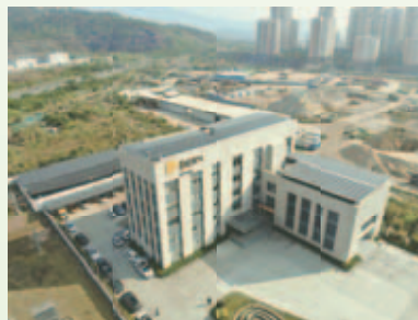
零碳場站現場 The site of zero-carbon station
